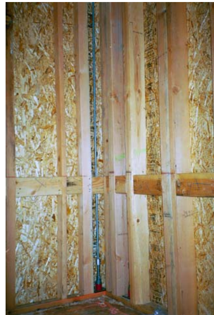
Adaptable building: Blocking in a bathroom wall for grab bars
