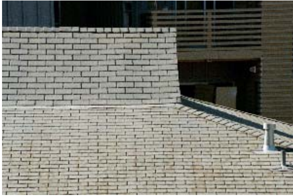
Community Center roof features recycled “fake-slate” shingles
