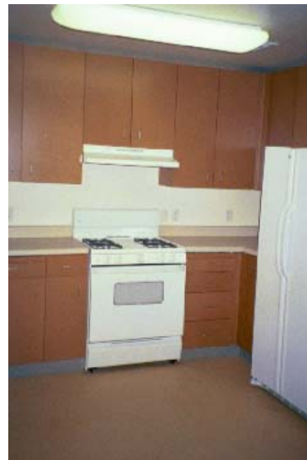
Kitchens feature natural linoleum, formaldehyde-free MDF cabinets, and ENERGY STAR ® appliances
