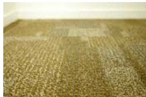
Carpets are made of recycled and recyclable material, laid in tiles for easy maintenance
