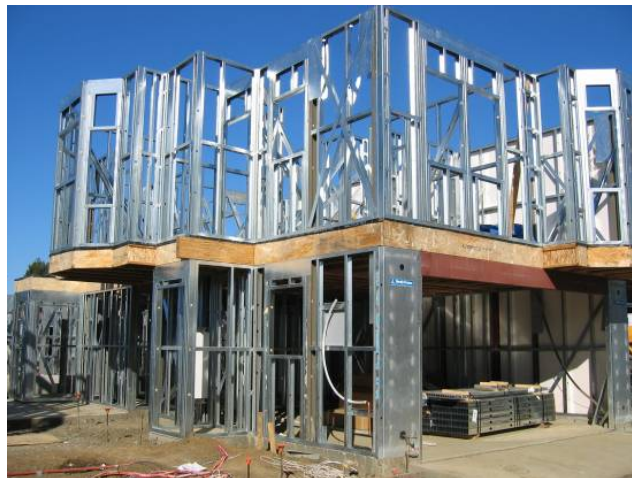
The steel framing of a Phase II unit
