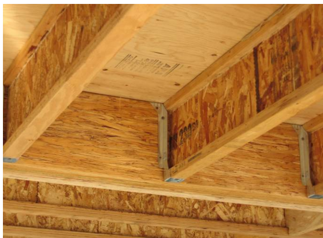
MCM chose resource-friendly engineered lumber over dimensional lumber for the joists and beams.
